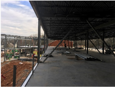
Elevated Deck & Roof Decking
