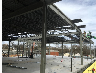
Elevated Deck & Roof Decking
