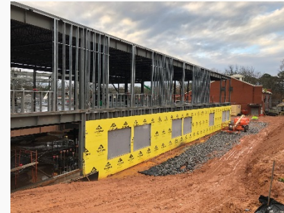
Exterior Framing & Sheathing
