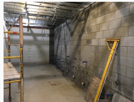
Masonry Chase Wall at Restroom
