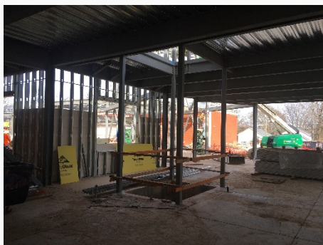
Elevator Pit and Frame
